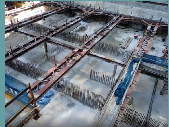
9000m<sup>3</sup> 3-metre Thick Raft Foundation, CPF Tower (2018)
